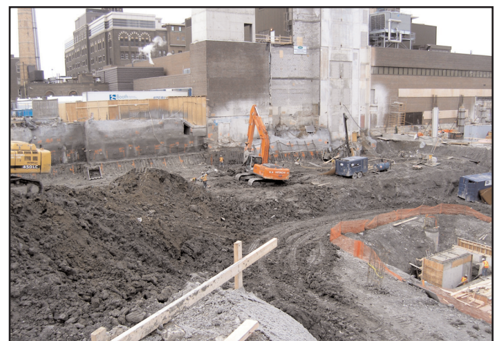
Pictures show the redevelopment project taken March 28, 2008
